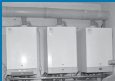
Central Baxi high efficiency boiler plant
