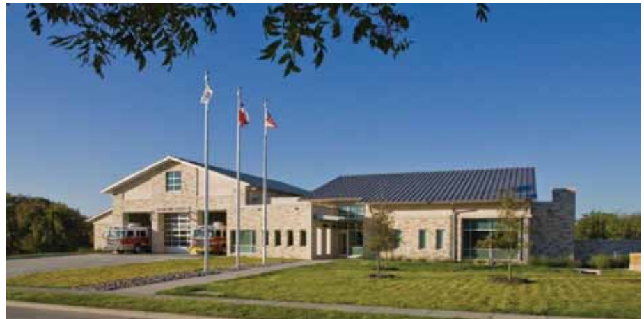
The 15-ton heat pump installed at Plano (TX) Fire Station No. 13 offers the opportunity to test the operating costs of gas vs. electric cooling. Energy use and cost at the station will be compared with that of another "twin" station using electric cooling technology.
